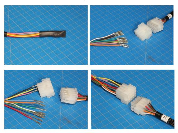
If you install the wire in the wrong hole, slide the provided tool into the connector, while pushing in on the wire to get the barbs away from the housing, wiggle the removal tool onto the terminal, when set pull the wire out and install in proper hole
